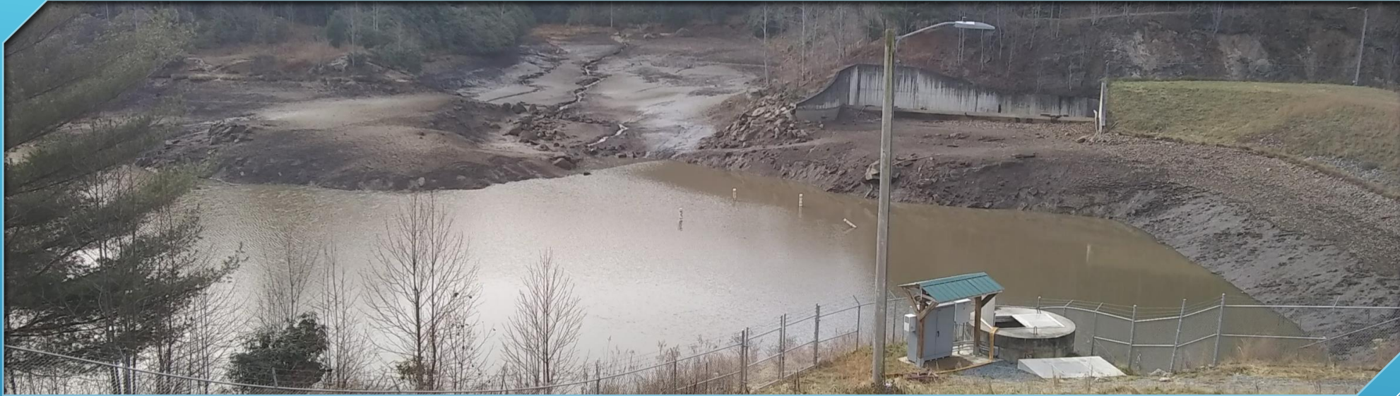
Buckeye Lake Reservoir November 2018
