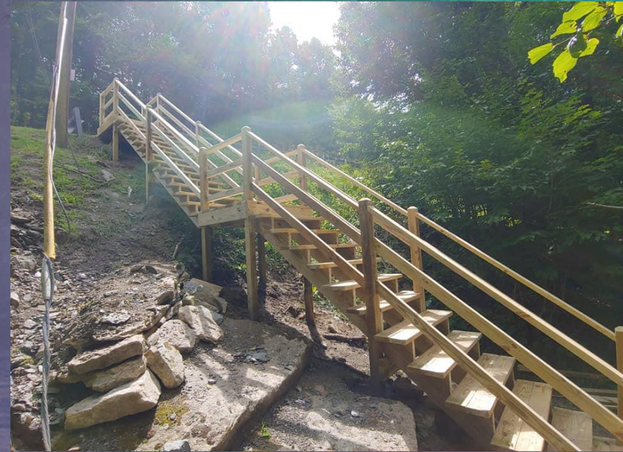
Upper Pond Creek Stairs
